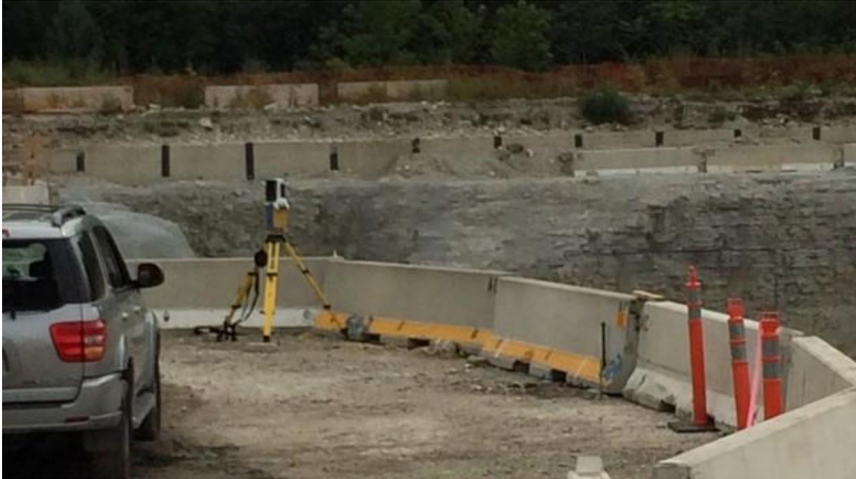
*Contractor J.J. Henderson used a robotic total station to set control points throughout the site as a basis for registering their 3D laser scanner point cloud data.*
