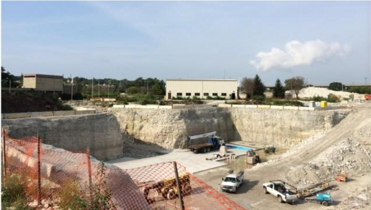
*The new wet weather reservoir and wet well is a large in-ground concrete structure that measures 215 by 165 by 30 ft. deep. The concrete walls are 2.5 to 3 ft. thick, and the base measures 4 ft. thick.*
