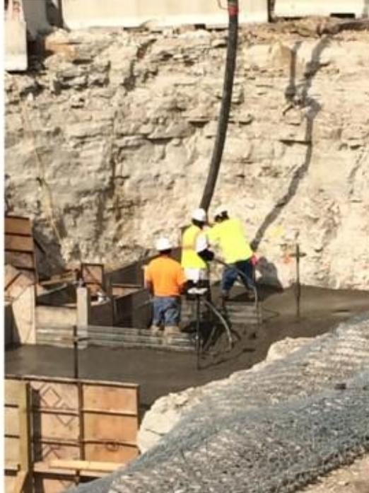
*The construction of the concrete wet weather reservoir structure began with pouring a 1-ft. thick mud slab as a level footing for the base slab varying between 3 and 5 ft. in thickness.*
